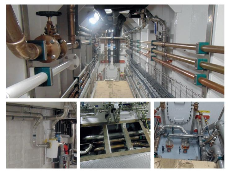
Pendennis Shipyard, said: "Boat piping installations are often complex due to the lack of straight lines. Geberit's Mapress system simplified this challenge. The press-fit method ensured secure connections, reducing errors during installation.
